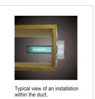
AirScrubber Plus can be installed in any HVAC system directly into the ductwork or directly above the air handler in remote or "down stream" locations.
